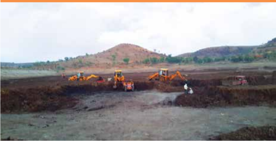
River Rejuvenation work conducted by local community and NGOs at Beed district supported by Capital First
